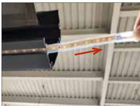
10. Pull the LED strip out of the groove in the front bar slowly.
