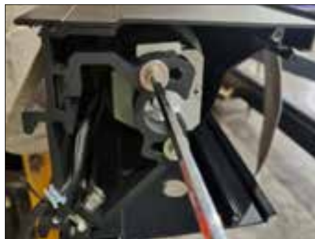
8. Use the same tool to remove the screws connecting the motor to the roller bracket.
