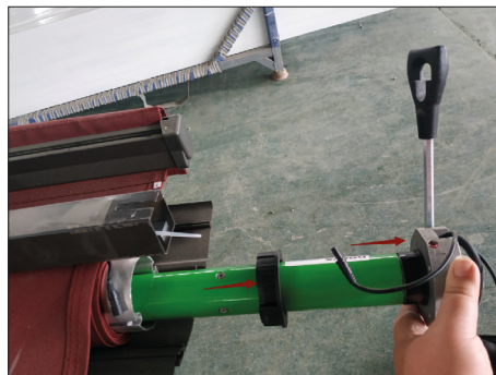
11. Pull the motor out.
