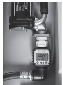
Fig. 6.2.2: Flow meter for 4301 / 4601 / 6001 tank
