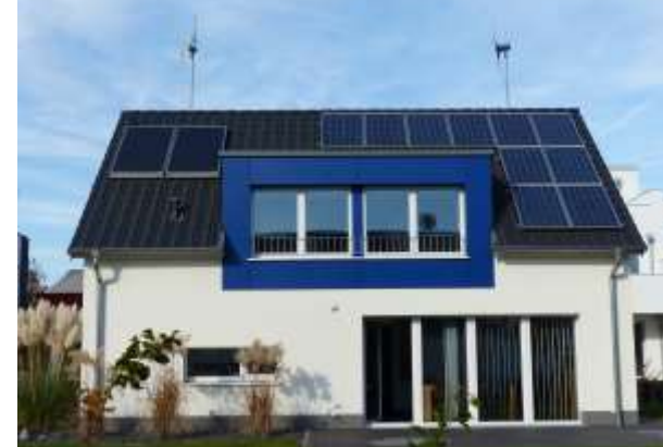
Decoupled towers mounted under the roof-tiles
