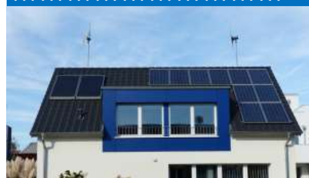
Mounted on a standard rooftop
