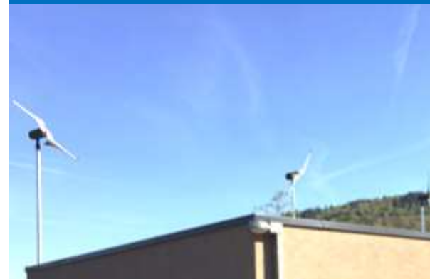
Flange-mounted to a flat roof building
