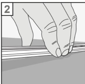
2. Place the profile on the floor in the desired position, and press down hard.
