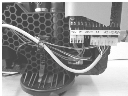
Fig. 7: Insert plugs A1 und A2 into ports of control unit
